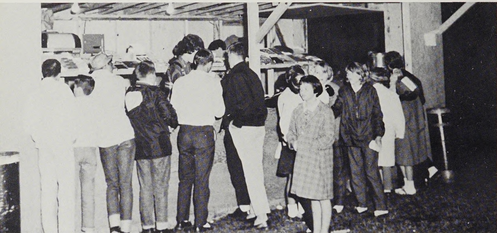
The newly constructed concession stand, another project of the Key Club, takes in needed money for school projects.
