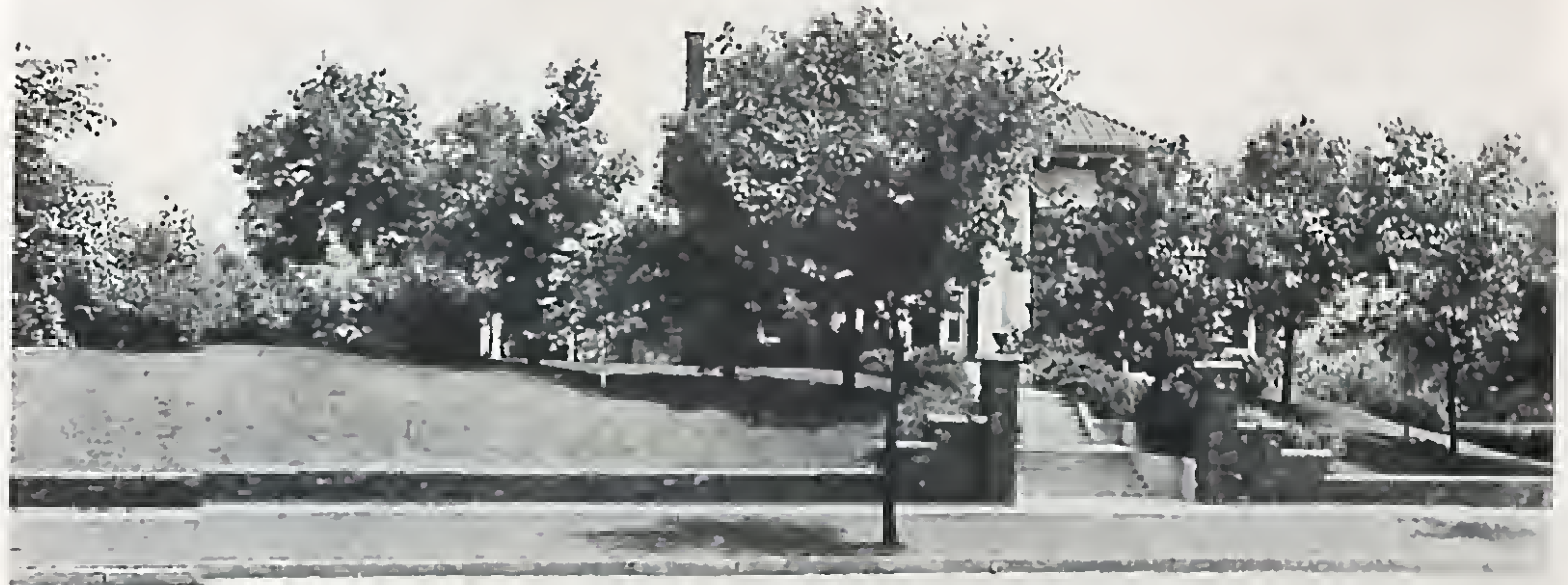
A well planted place showing a large open lawn
