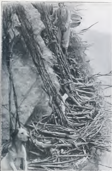
"THE NATIVES CONSTRUCT HANGING GALLERIES OF BIRCH TWIGS AS 'HIGH ROADS.'" (the Author.) From a Photo. by
