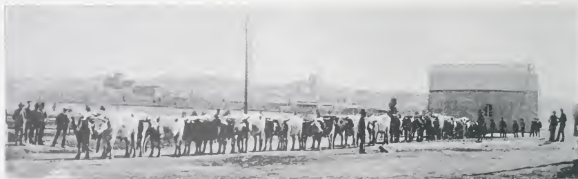
LARGE STORE REMOVED BODILY NEARLY TWENTY MILES BY A TEAM OF BULLOCKS.
