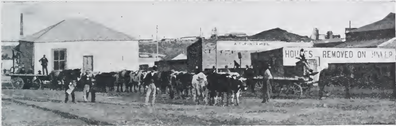
HOUSE-MOVING IN BROKEN HILL. A PRIVATE RESIDENCE BEING SHIFTED. From a Photograph.
