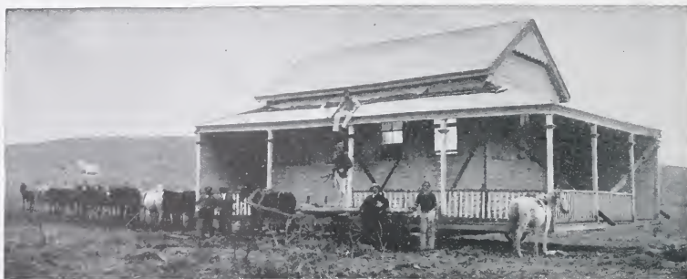
"THE PROGRESS OF EDUCATION"—A PUBLIC SCHOOL BEING "JINKERED" (WEIGHT 25 TONS). From a Photo. by Devon Photo. Company, Broken Hill.
