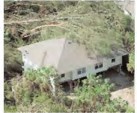
Mature Casuarina trees reach heights in excess of 100 feet. This means that when they do topple, their massive surface area tends to have a greater impact on surrounding vegetation and structures.
