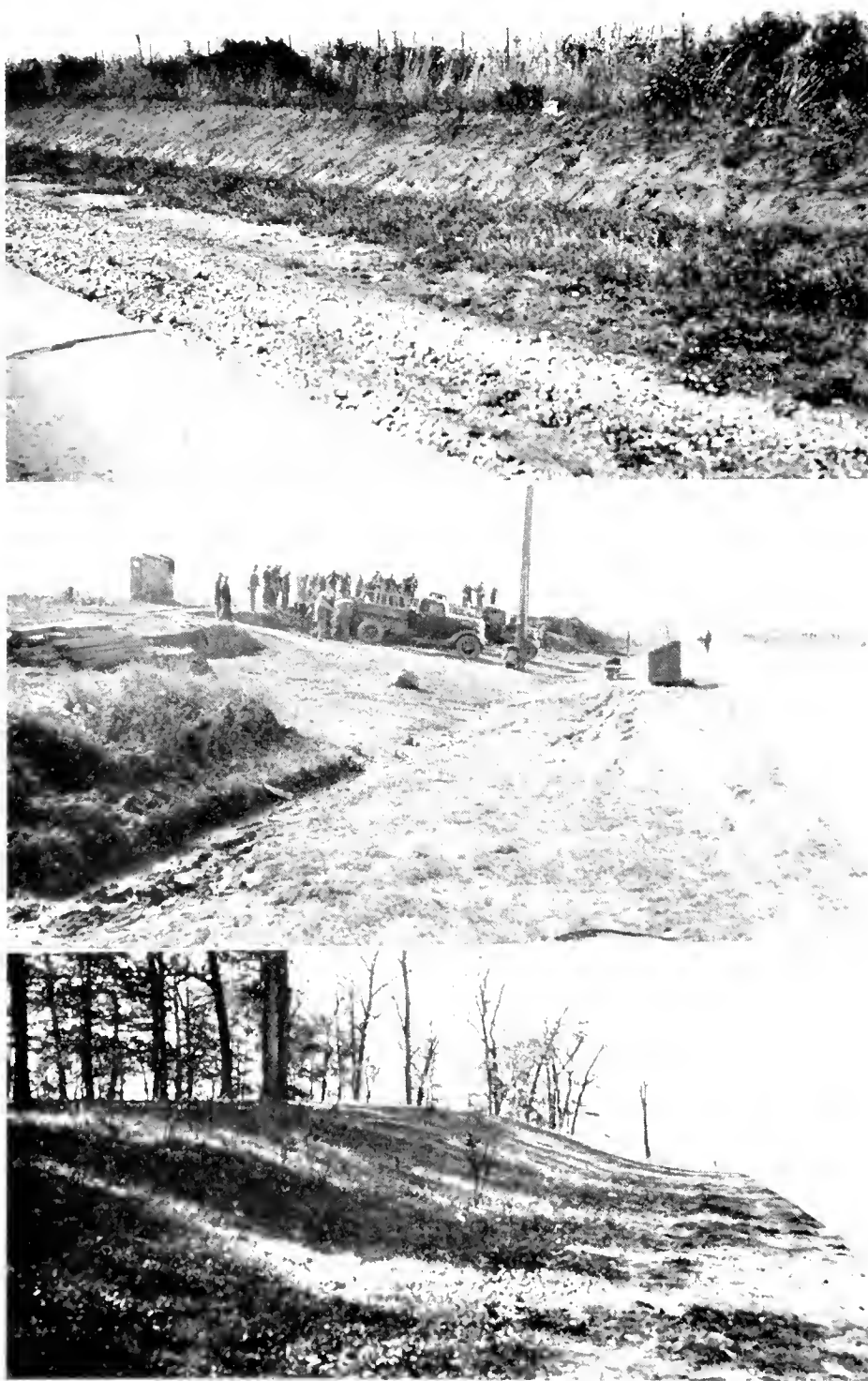
FIG. 18. Showing artificial changes in road margins. Top, example of original roadside condition; middle, showing the C.C.C. crew sloping the bank preparatory to planting; lower, a finished piece of roadside, after it has been graded and planted.
