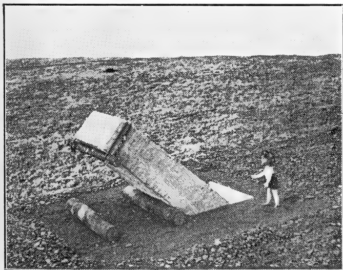
Fig. 2.—The upright tipped into the foundation pit.
