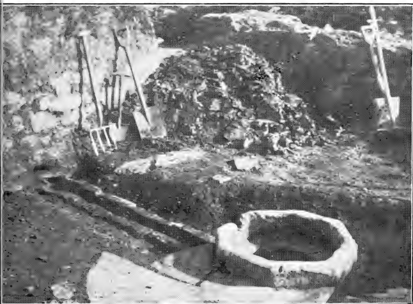
PLATE I.—Two views of Basin and Drain in floor of Room in Roman Villa at Nuthills.
