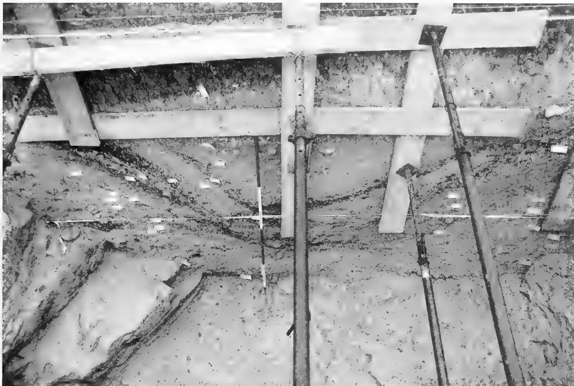
Plate 3. The east side of Inner Ditch North in Trench B, from the west. Scale in m
