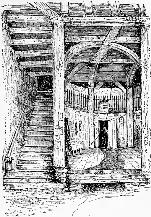
INTERIOR OF THE CURFEW TOWER
