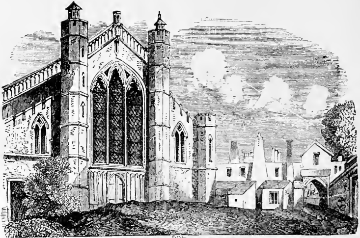
WEST END OF SAINT GEORGE'S CHAPEL
