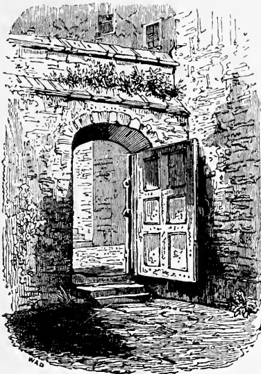
OUTER DOOR LEADING TO THE HUNDRET STEPS
