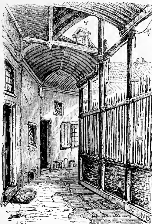
PART OF THE HORSE SHOE CLOISTERS
