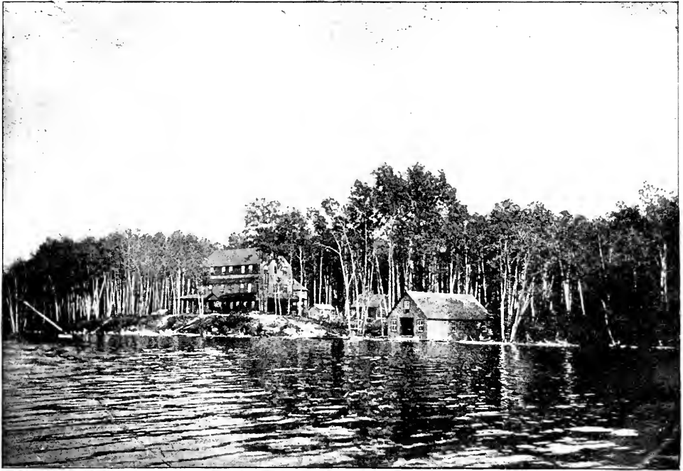
MEGANTIC CLUB BUILDINGS, MACANNAMAC LAKE.
