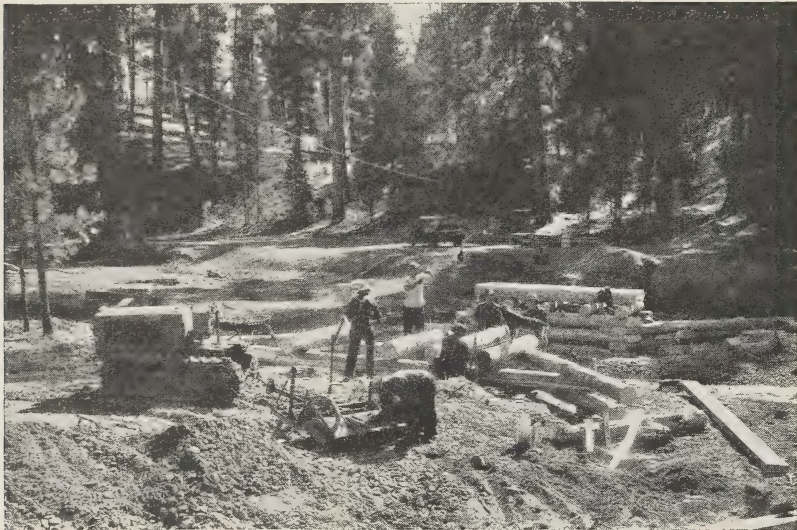
FIGURE 14.—Crew constructing buttress for bridge across Elder Creek in the Fremont National Forest, Oreg.
