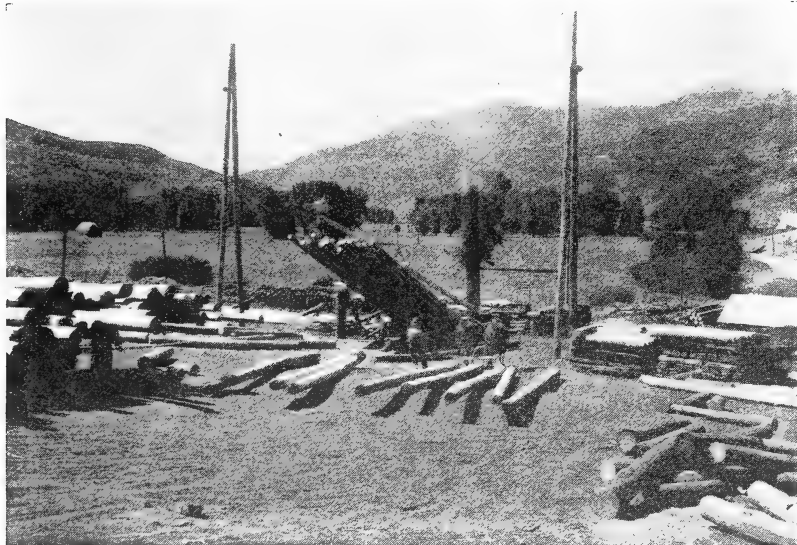
FIGURE 24.—Treating poles from the Wasatch National Forest, Utah.
