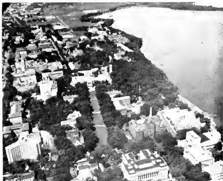
UNIVERSITY OF WISCONSIN CAMPUS, WITH HYDROBIOLOGICAL LABORATORY IN THE LOWER RIGHT HAND CORNER
