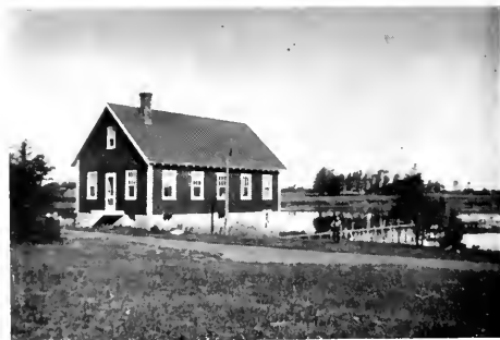
BIOLOGICAL SUB-STATION, ELLERSLIE
