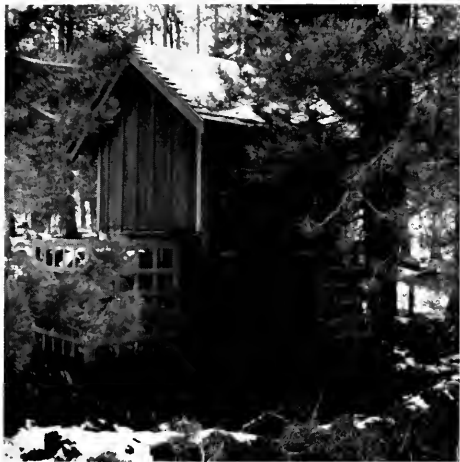
UNDERWATER OBSERVATION TANK, SAGEHEN CREEK EXPERIMENTAL WILDLIFE AND FISHERIES STATION
