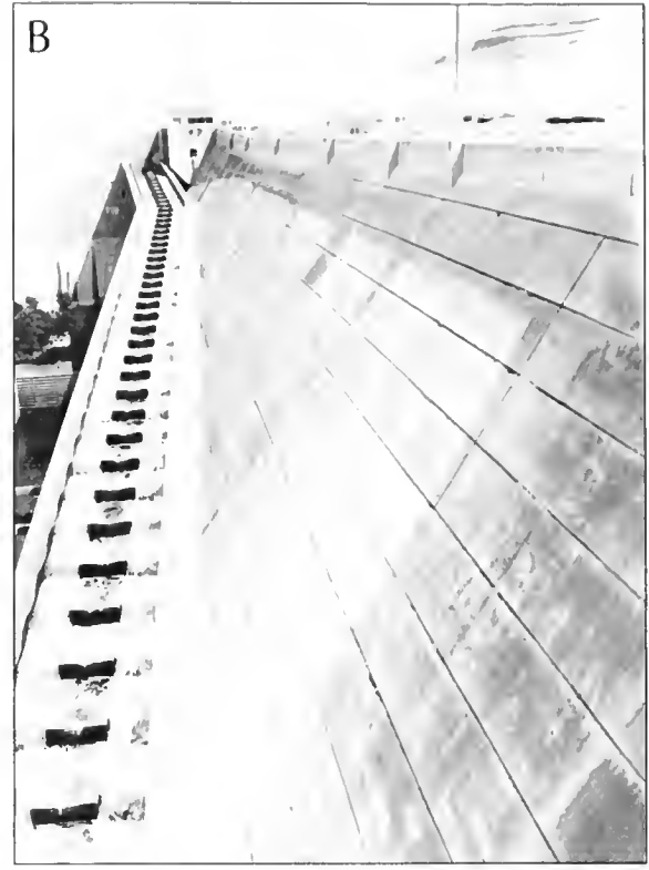
Fish ladders at one of the eight federal dams salmon must pass to reach Idaho spawning grounds. Lower Monumental Dam (Bonneville Power Administration)
