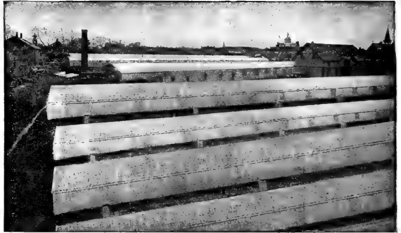
The above illustration shows only a small portion of our plant.
