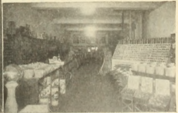
Retail Seed Store with Main Offices in Rear
