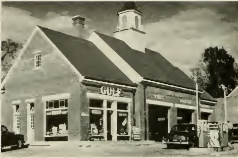
Phillip Andrews Service Station • Chapel Hill, N. C.
