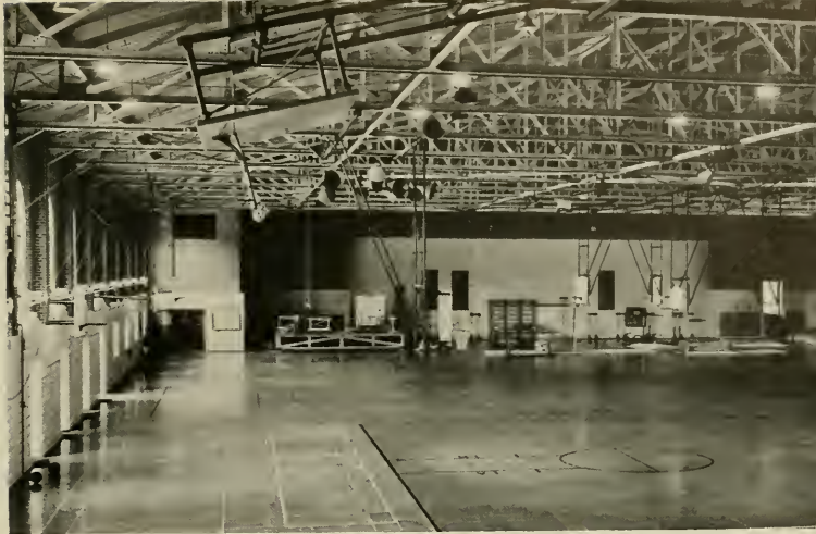
A portion of the 250 by 150 feet Woollen Gym floor (above) may be converted into an indoor track or eight complete basketball courts. Note adjustable backboard at top left.
