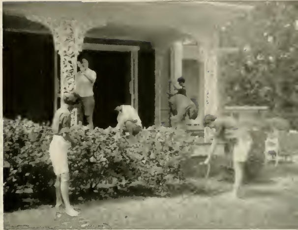
Tri Deltas make repairs.
