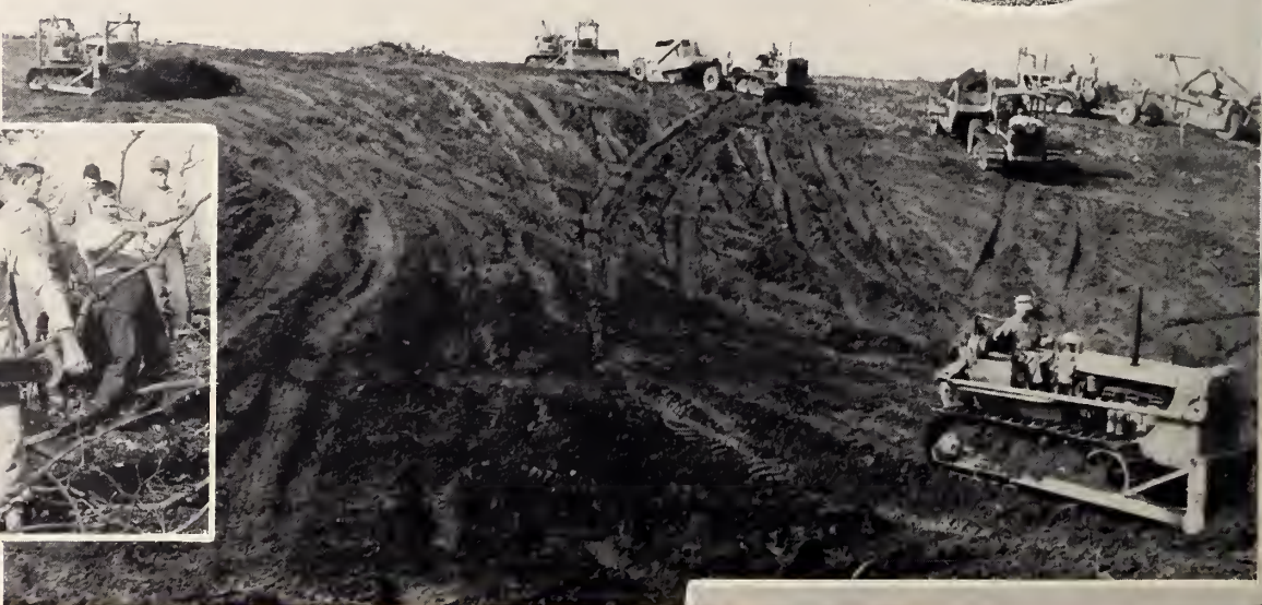
Bulldozers and pans on the move.
