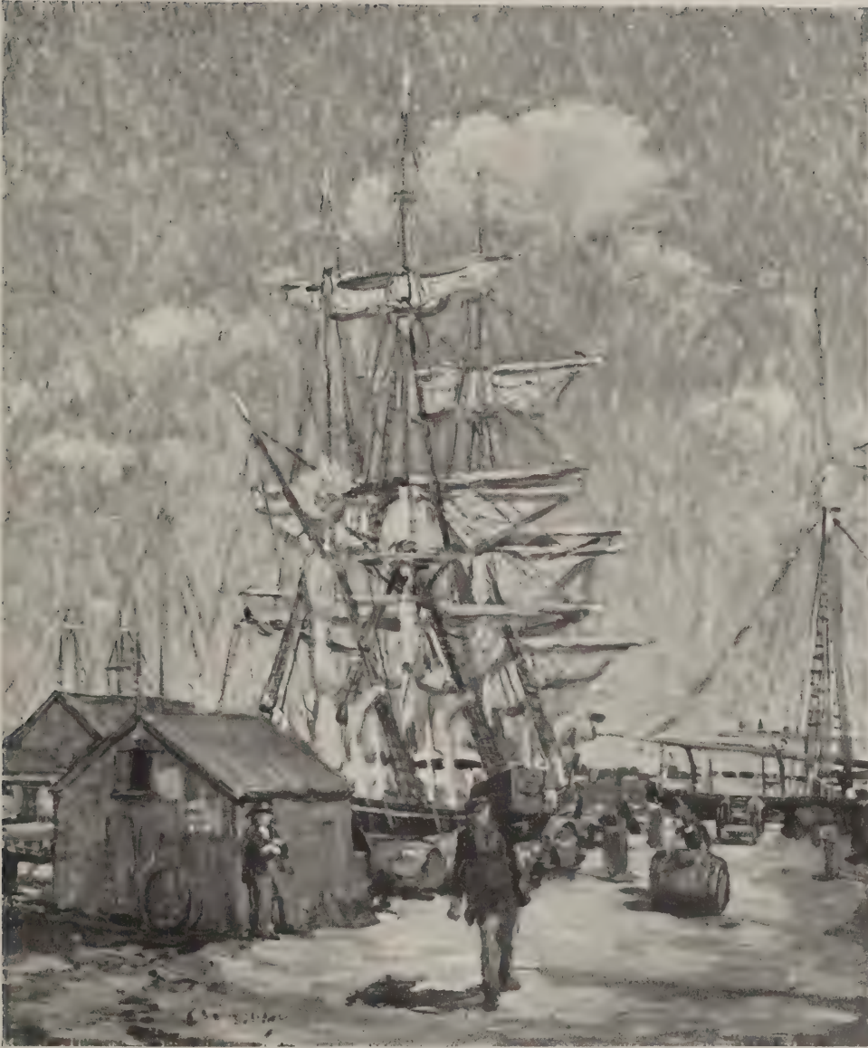
THE WANDERER WITH SAILS CLEWED Breaking out oil
