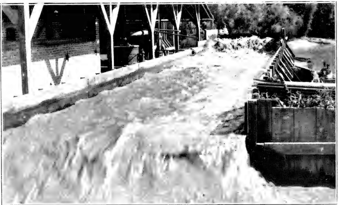
FIG. 2.—PUMPING PLANT FOR RICE IRRIGATION.
