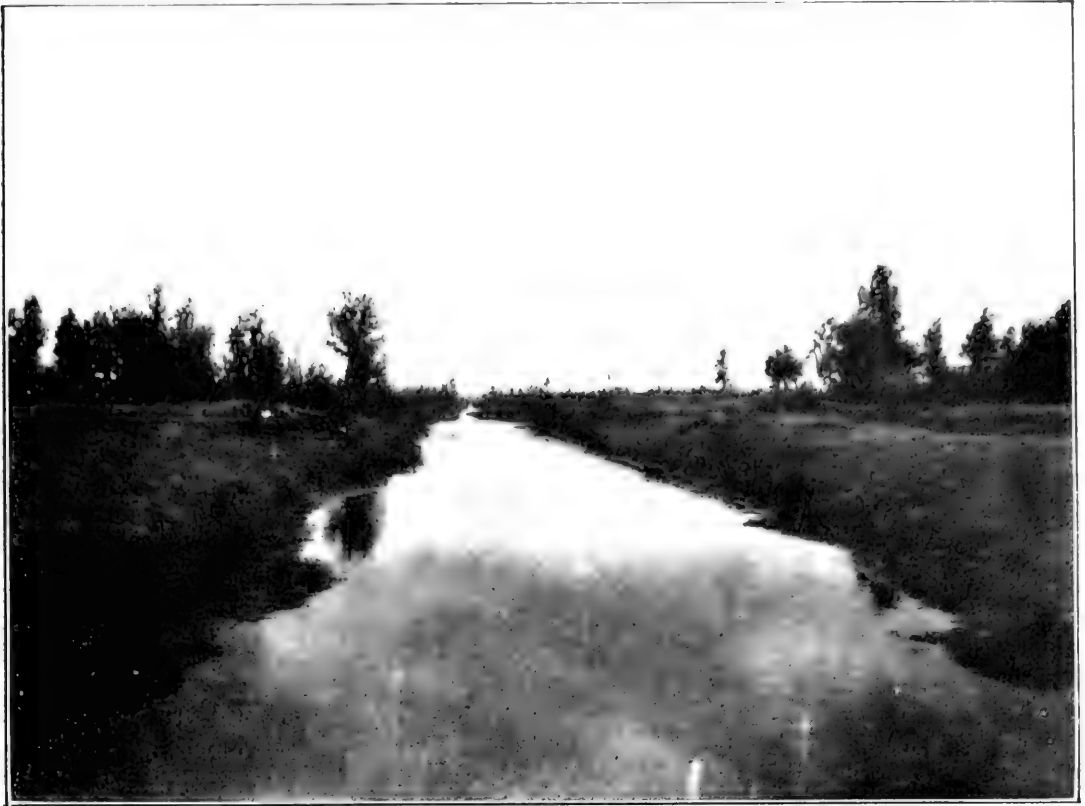
FIG. 1.—CANAL USED AS RESERVOIR, CRANMOOR, WIS.
