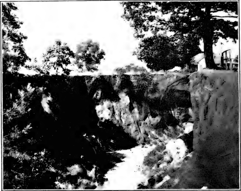
FIG. 1.—EROSION IN COASTAL PLAIN UPLANDS.
