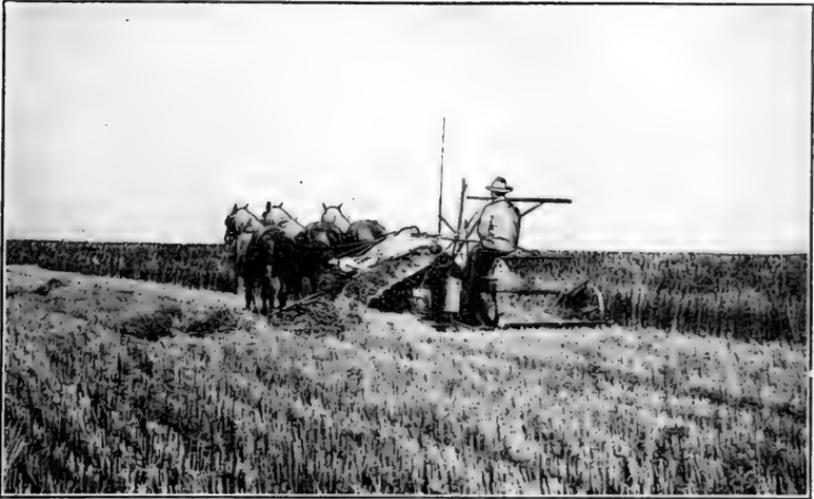
FIG. 1.—SELF-BINDER IN OPERATION.
