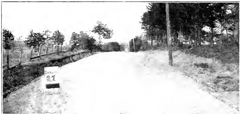
FIG. 3.—FINISHED MACADAM ROAD.
