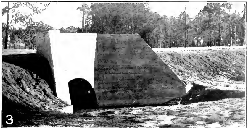
FIG. 3.—CONCRETE BRIDGE, TEXARKANA, ARK.
