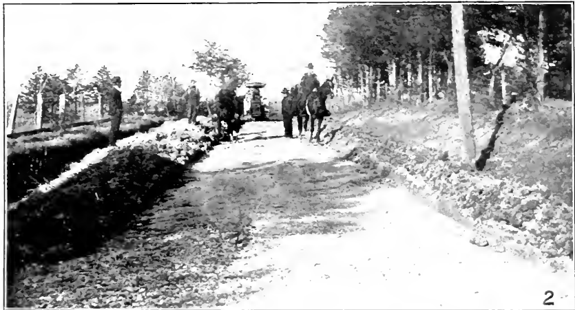
FIG. 2.—SUBGRADE READY FOR MACADAMIZING.
