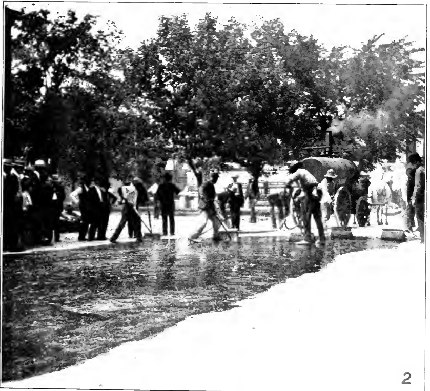
FIG. 2.—TARRING ROAD AT JACKSON, TENN.—LATEST ADVANCE IN ROAD SURFACING.
