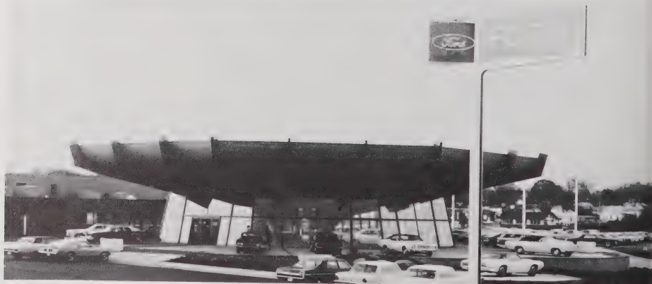
laminated beams and roof decking for the sanders ford company bldg raleigh nc (pictured above) manufactured and furnished by koppers company inc morrisville nc
