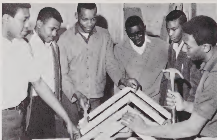
Carpentry students at West Cary watch as Danny Pearson begins hammering once again on their dog-house.
