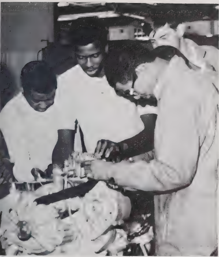
Kelly Gist watches as Malone Carrington demonstrates to Eddie Rich and Calvin Bledsor how to adjust the valves on an automobile engine.
