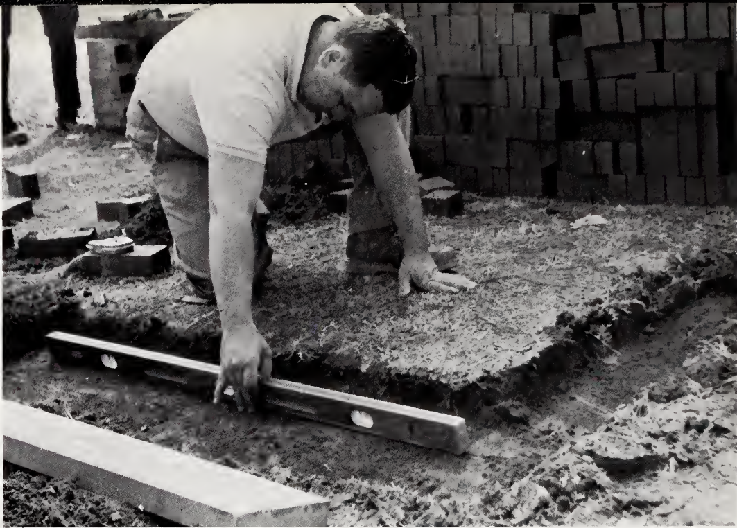
Robert Hoyle is using the plumb rule to make sure the corner is level before erecting a broken bond corner.
