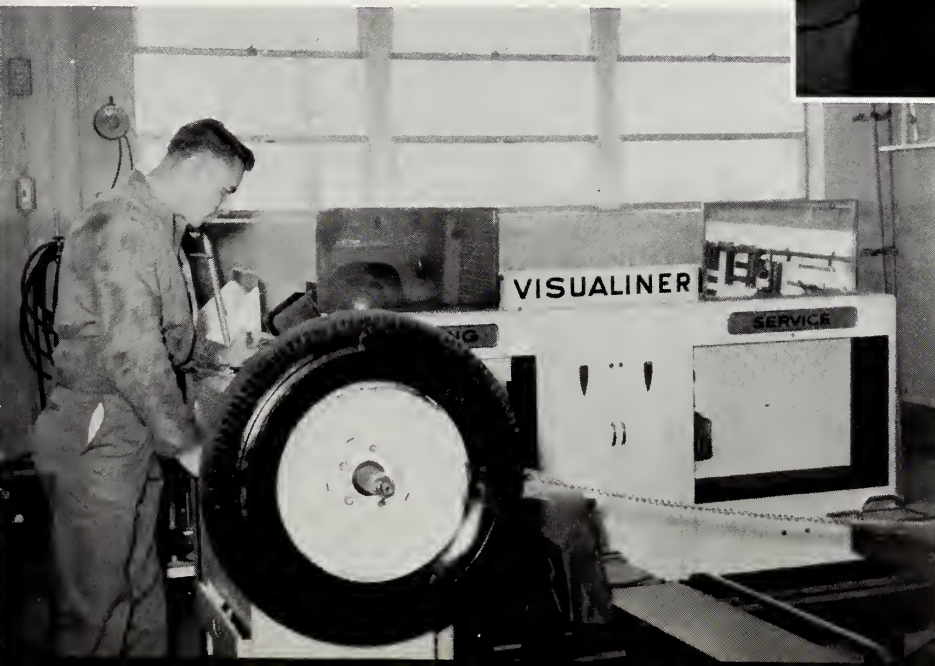
Lonnie Whaley is balancing a wheel with the electronic balancer.
